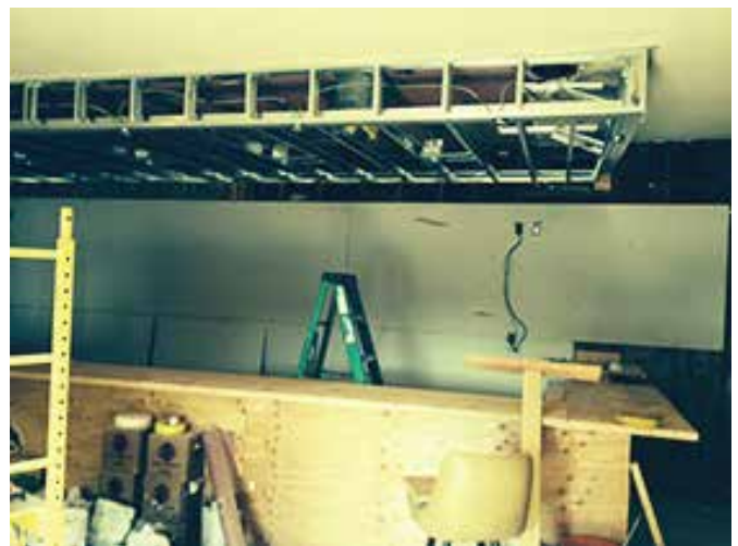
More Pics of Lounge Renovation
