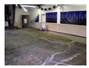
Lodge room floor in progress-cracksfilled---laminate floor to be installed
