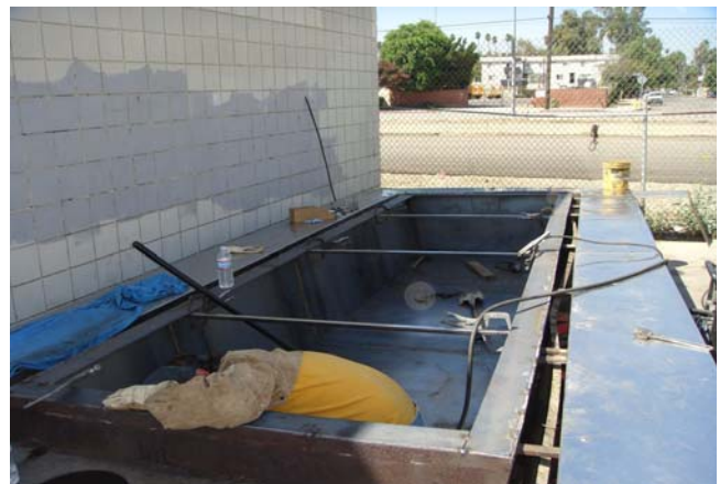
BBQ A Work In Progress a new firebox
