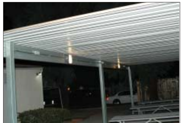
Notice the addition of illumination installed by the Grunts to enhance our outdoor patio on warm summer nights.
